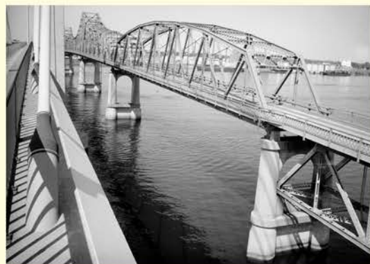
The historic Green Bridge (right, 1922–1978), stands beside its modern successor, the Ed Hendler Cable Bridge (left).
