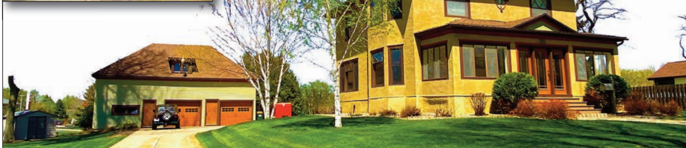
The Dowling residence and Carriage House are in terrific shape thanks to the property's various owners during its over century old existence. Located on Depue Ave. in Olivia, recent initiatives have explored acquisition of the home due to its potential to serve the community and Yellowstone Trail tourists.
