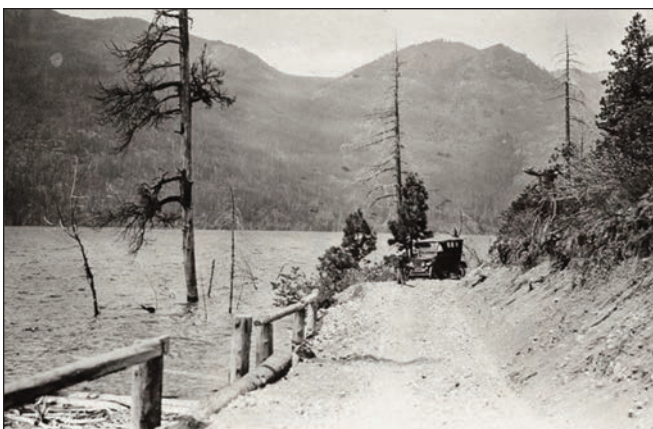
A photo of the Yellowstone Trail road over Snowqualmie Pass in Washington in 1915.
