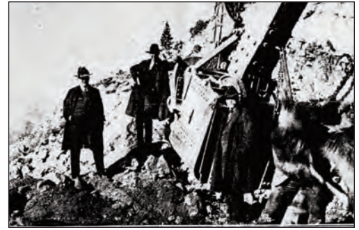
A big steam shovel at work on the Davis Grade in 1921.
