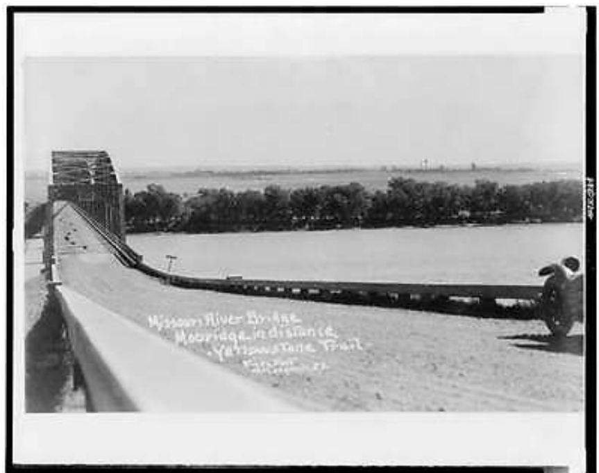
1924 Missouri River Bridge on the Yellowstone Trail looking East to Moberge
