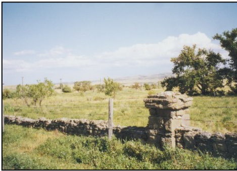
Only this Stone wall and spring remain
