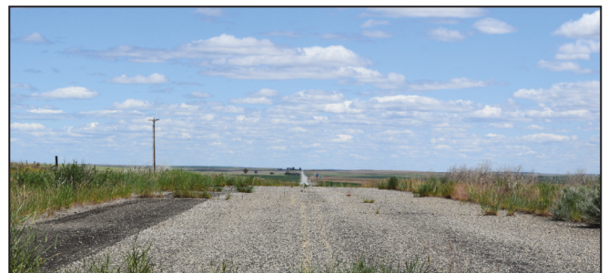
Old Road Eastbound from Waterville, Washington
