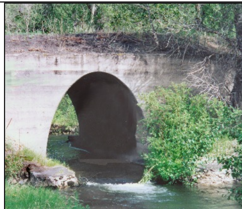
Fridley Creek Bridge
