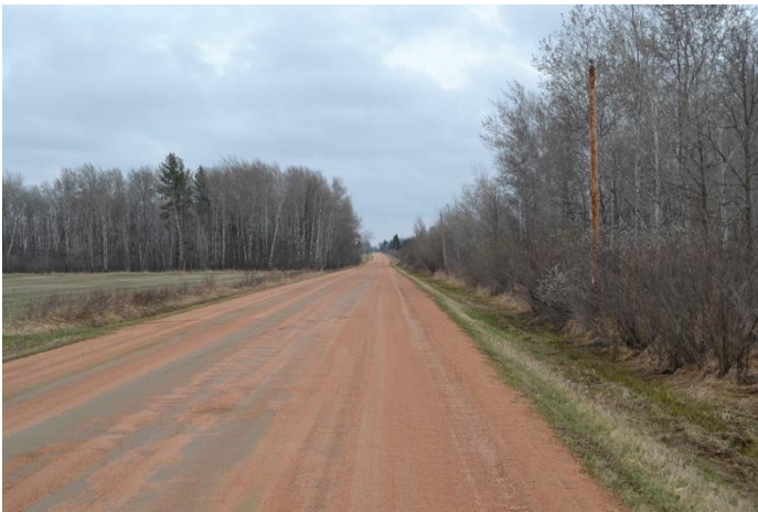
Elm Road West of Stevens Point, Wisconsin
