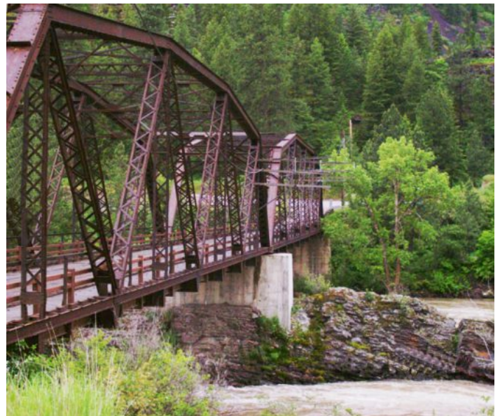
The Natural Pier Bridge near Alberton, Montana. It makes use of the rock outcropping in the center of the river.
