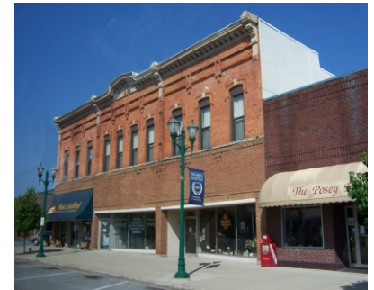
These buildings in Hicksville, Ohio, look pretty much the same today as they did to a Trail traveler in 1920.
